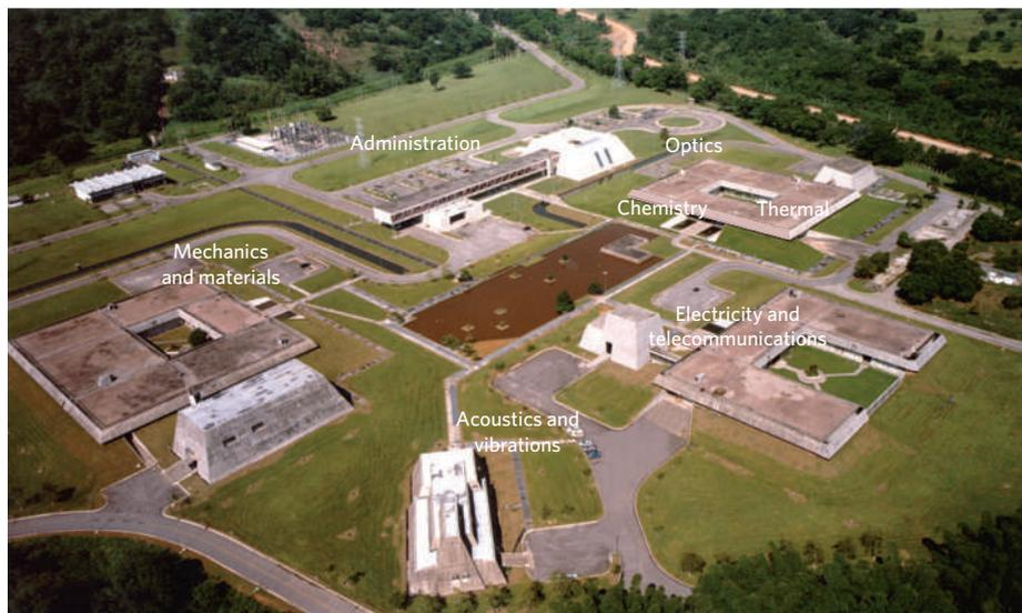
**Figure 4** | Part of the scientific campus of the Brazilian Metrology Institute (Inmetro). The campus is based on a special geological area and far from any urban centre. Most laboratories are built on top of concrete, rubber and sand, without physical connections with neighbouring laboratories and corridors. Picture courtesy of Inmetro.
